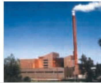
Heimdal heating station
