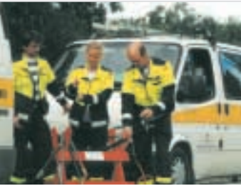
Cable installers working on the grid
